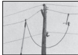
Install other end of jumper on conductor.
