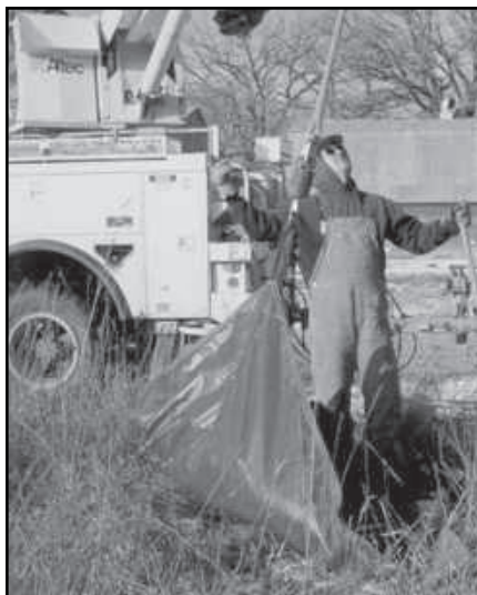
Winching TWISTARP with truck for filling.
