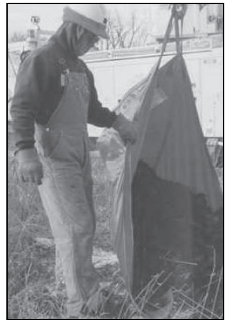
Dumping TWISTARP with winch to fill hole.
