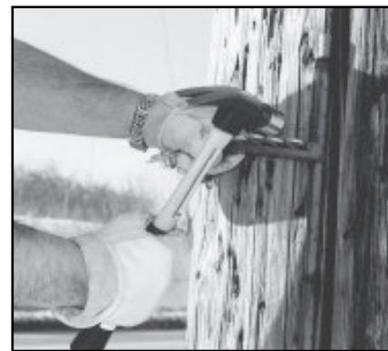
Hold the stick with staple over the ground wire, hammer top of staple to get started, pull staple stick away and set staple.
